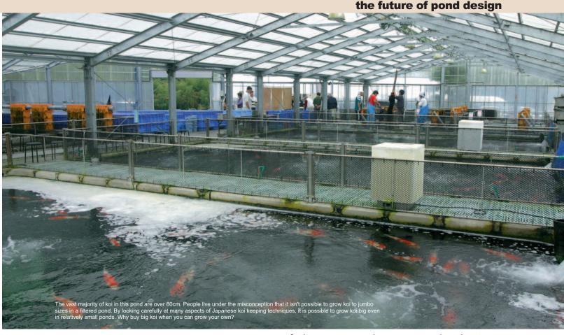
The following is an overview of a pond that I have designed for a customer here in the UK using Mr Maeda's design principles. The pond will contain around 10,000-gallons, of which almost the entire footprint consists of pond space, not filter space. By doing this, it has been possible to design a pond that with conventional filtration, would have perhaps only contained 6,000-gallons (excluding filters).
